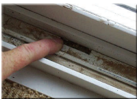
Interior Window Track should be cleaned and lubricated
